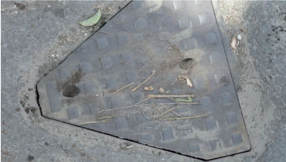
The arrow head shaped sewer covers show where the main channels are situated and in which direction it flows.
